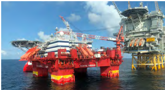
Floatel Superior commenced operations for Equinor Martin Linge project end-July 2018.
