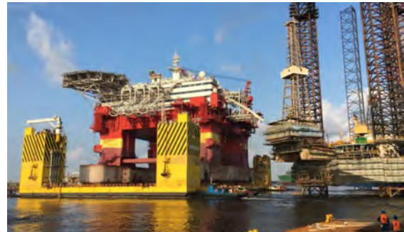
Following completion of rectification work and SPS Floatel Endurance left Singapore for Norway 19 July 2019.
